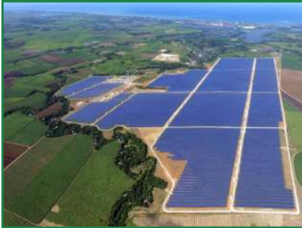
132.5MW Helios Solar Farm Cadiz City, Negros Occidental, Philippines
