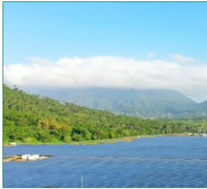
120MW Alaminos Solar Plant Alaminos, Laguna, Philippines
