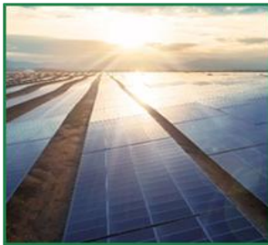
405MW Ninh Thuan Solar Ninh Thuan, Vietnam
