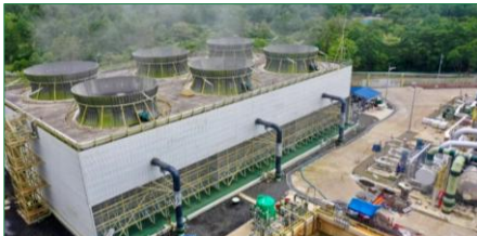
28.9 MW Palayan Bayan Binary Project (Steamfield), Albay
