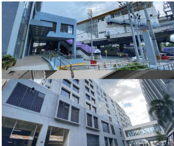
Sta. Lucia Business Center (outside view)
