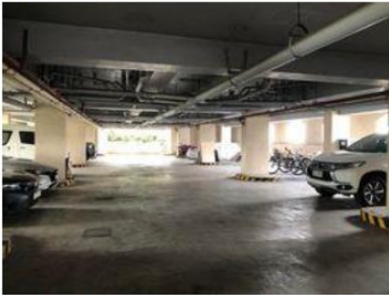
Parking at Lower Ground Level
