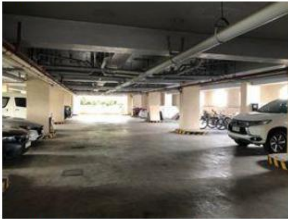
Parking at Lower Ground Level
