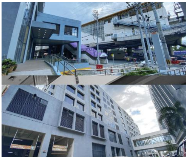
Sta. Lucia Business Center (outside view)
