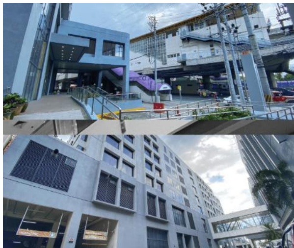
Sta. Lucia Business Center (outside view)
