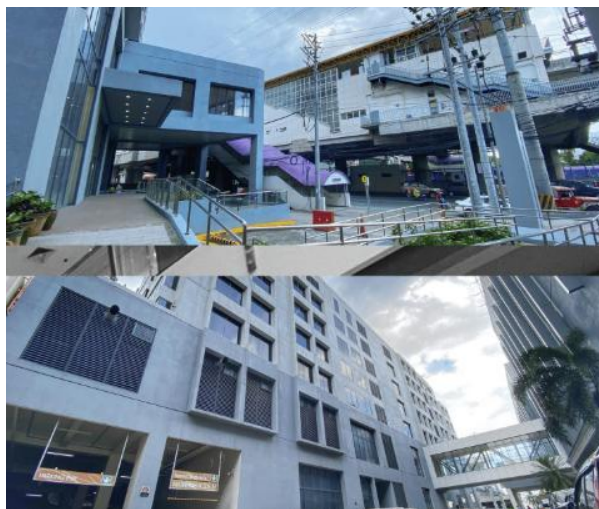
Sta. Lucia Business Center (outside view)
