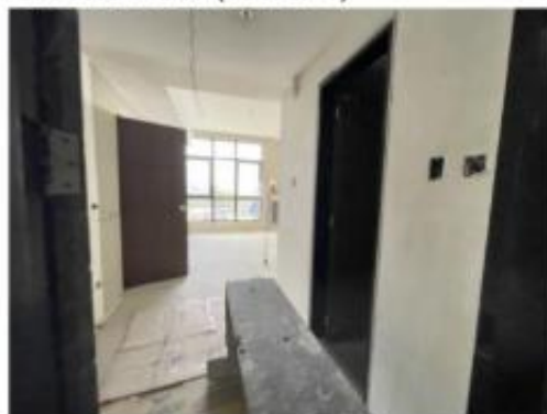
Sample Unit (Tower 1)
