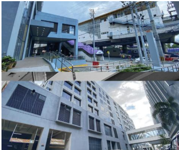
Sta. Lucia Business Center (outside view)
