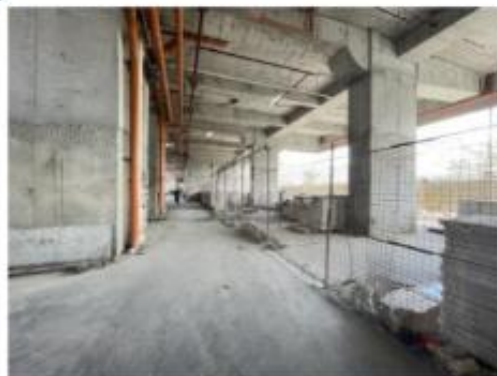
Ground Floor (Tower 1)
