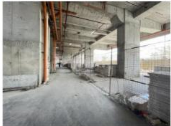
Ground Floor (Tower 1)
