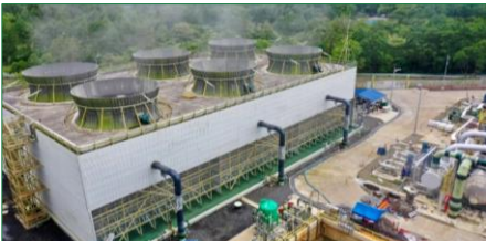
28.9 MW Palayan Bayan Binary Project (Steamfield), Albay
