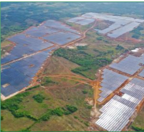
133MW Cagayan North Solar Plant Lal-Lo, Cagayan, Philippines
