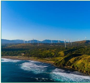
81MW N. Luzon Renewables Wind Pagudpud, Ilocos Norte, Philippines
