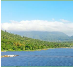
120MW Alaminos Solar Plant Alaminos, Laguna, Philippines
