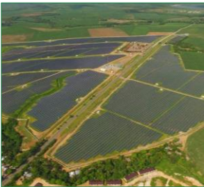
80MW La Carlota & Manapla Solar Plant Negros Occidental, Philippines
